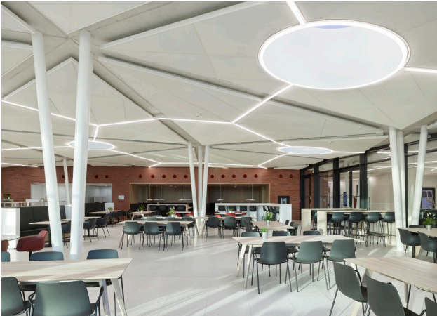
The light channel in the 'grid structure' cleverly integrates daylight from the skylight in the canteen.
